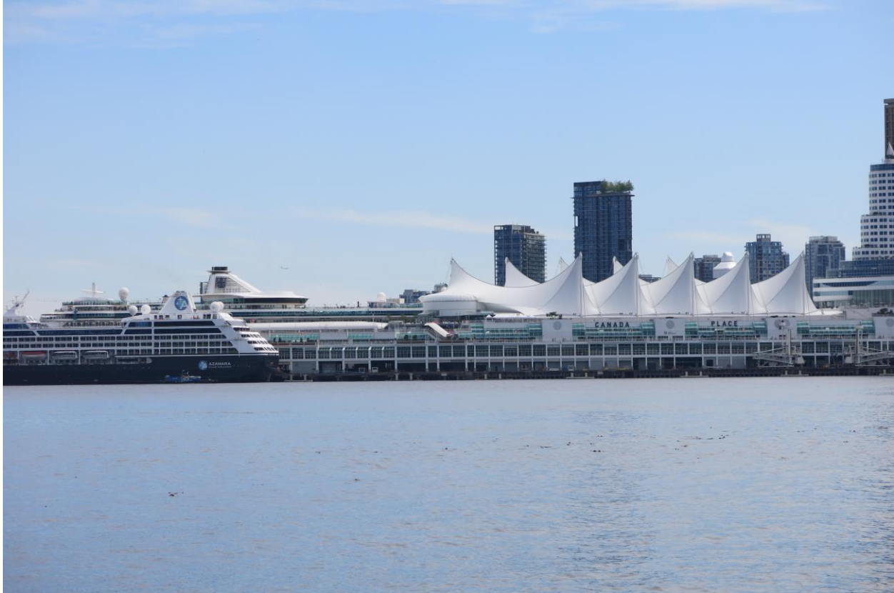
Figure 5. Cruise terminal - viewed from Stanley Park
