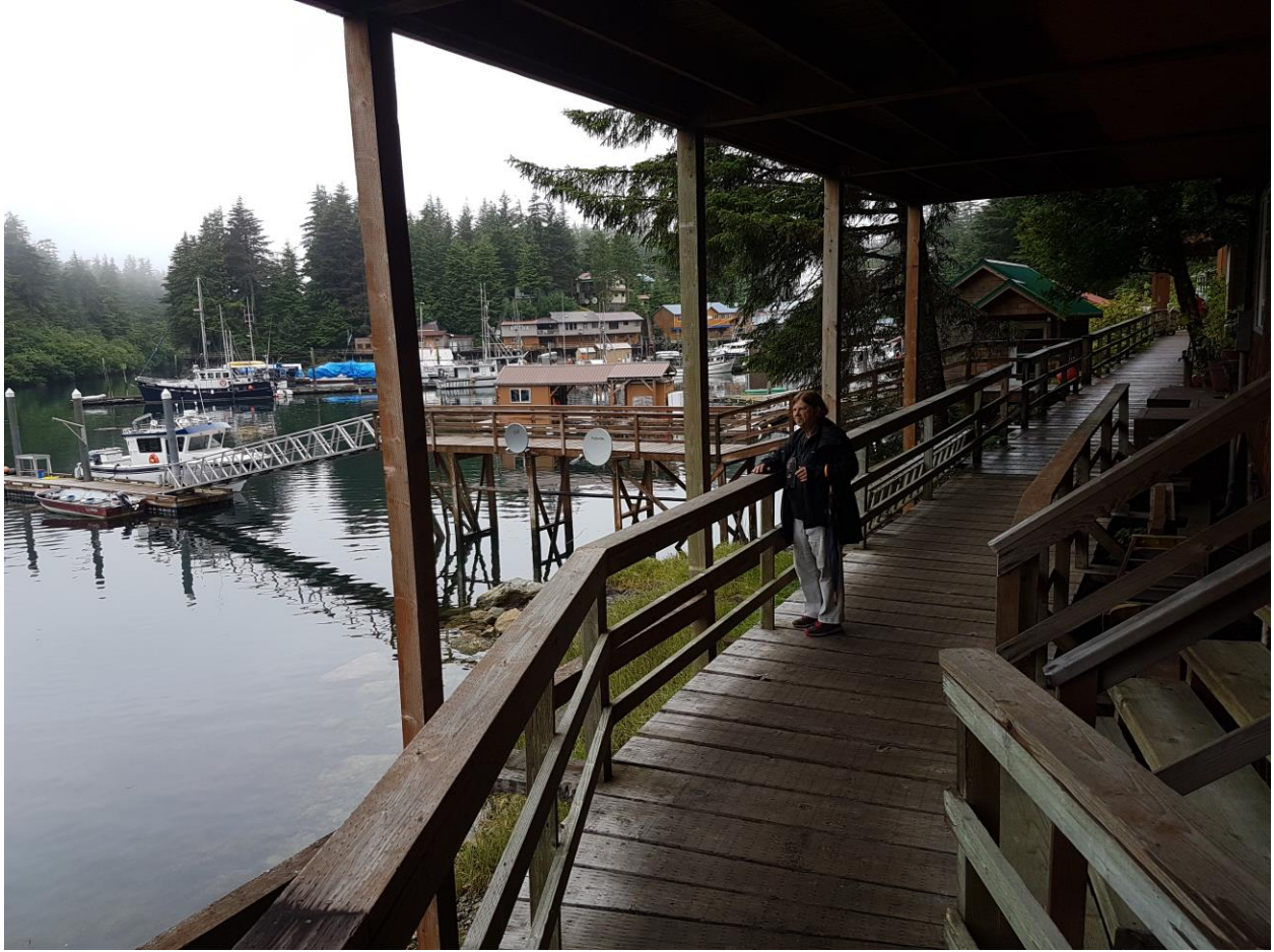
Figure 1. Boardwalk in Elfin Cove
